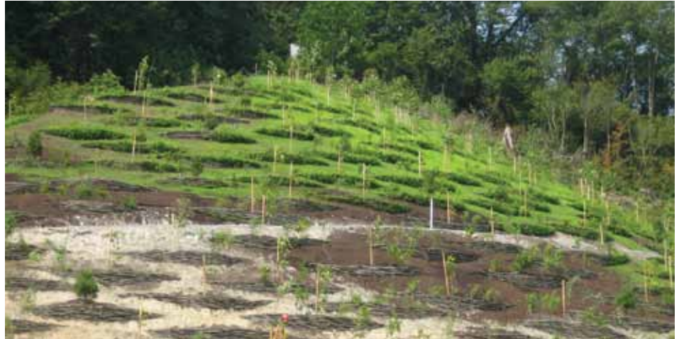
Environmental restoration efforts included the installation of over 300 wattles (for colour images visit www.sitelines.org ) Credit: Catherine Berris and Associates
